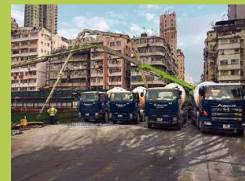
Concrete pouring at the project site 友盟混凝土車於地盤卸貨
