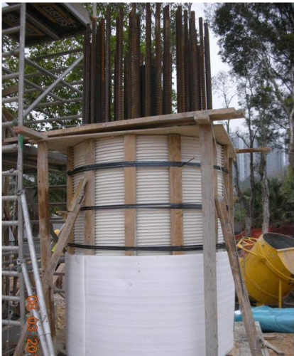
High strength concrete for column structure
