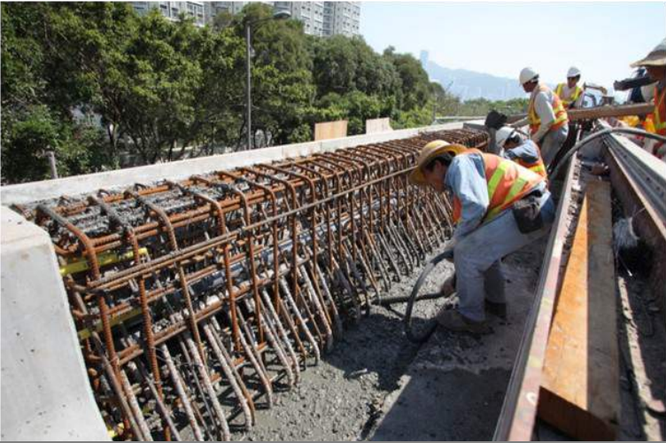
High early strength concrete to re-open the road within 6 hours for traffic
