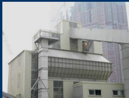
The fully enclosed production lines and materials delivery barge confined the transmission of pollutants to the surrounding environment and also isolated the noise generated from the machinery operations.
