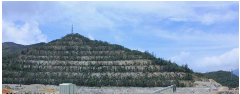
The completed bench at southern end of Lam Tei Quarry
