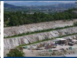
Completed bench at western side
