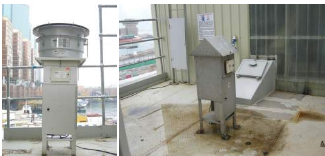
The air sampling devices we installed in the production plants monitor the TSP and RSP levels ensuring compliance to air quality standards providing useful data for evaluating the dust exposure of the surrounding sensitive receivers.
