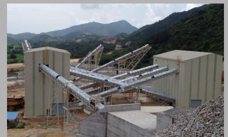
The fully enclosed crushing plant in our newly developed Huidong Quarry in PRC isolates the noise at its source
