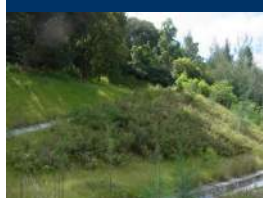
Completed slopes under close monitoring and maintenance
