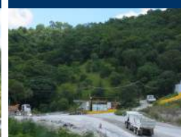
Completed rock filled slope at eastern side of the quarry
