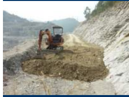
Formation of bench in progress
