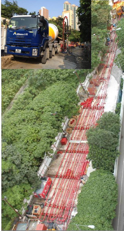
Concrete for long pipeline pumping
