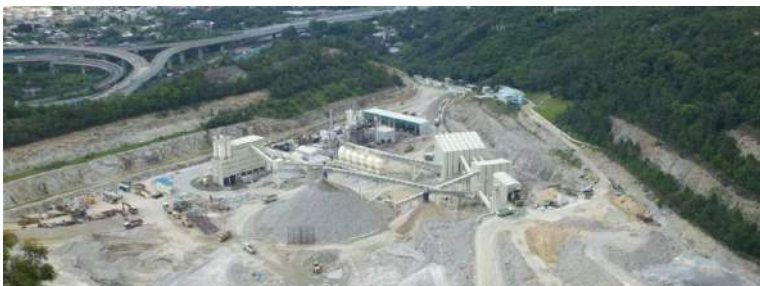
The quarry benches at Lam Tei Quarry barricaded the operation plants suppressed the transmission of noise and dust to surrounding areas.
