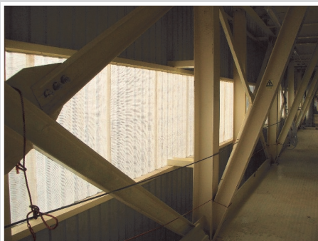
Translucent cladding to allow penetration of natural light
