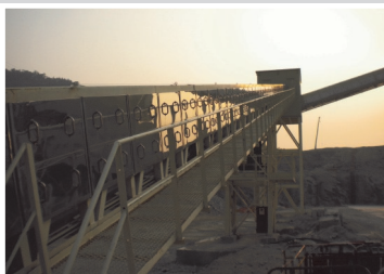
Conveying of aggregate is carrying out by dust tight conveyor system
