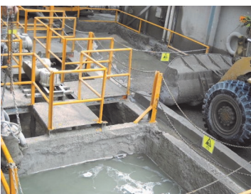
Coarse materials settled in the sediment pits before further treatment of the slurry water
