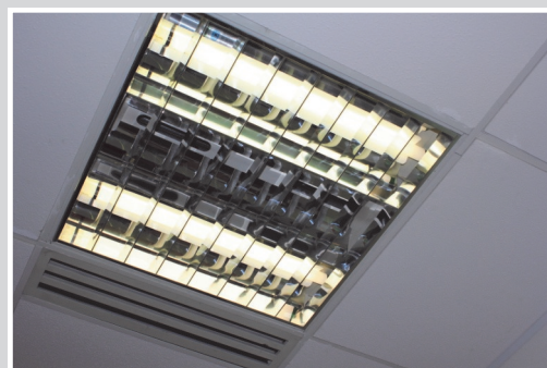
30% of Head Office's ceiling lights reduced after the installation of nano reflector
