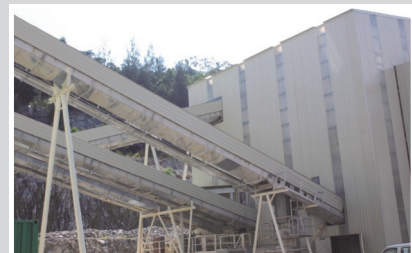
Noise and other pollutants are isolated in an enclosed structure
