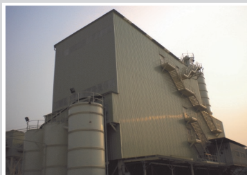
Noise and other pollutants are isolated in an enclosed structure
