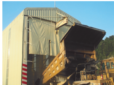
Dust emission suppressed by sprinkler system
