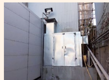
Cement pumping system was enclosed with G.I. acoustics panels and silencers for the natural ventilation
