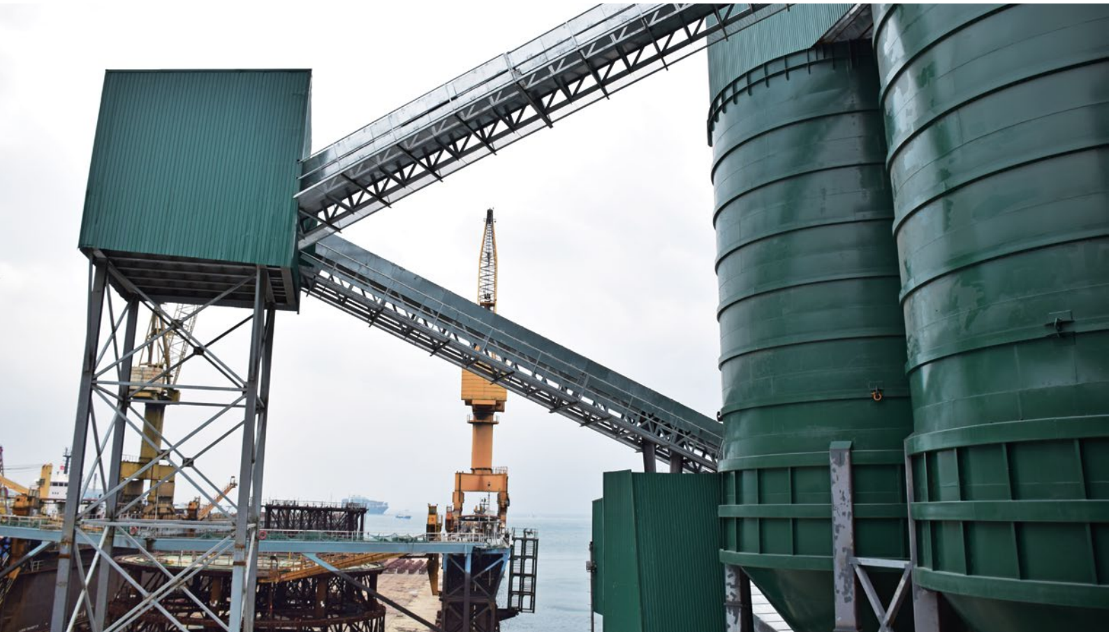
The enclosed structure isolated the emissions at their sources
