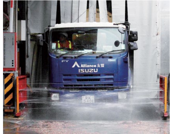
Trucks are thoroughly cleaned before leaving the site
