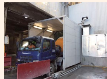
Mixer truck loading bay was enclosed with 100mm thick G.I. acoustics panel, not only reducing the noise impact to the environment site workers also benefit from the lowered noise level.
