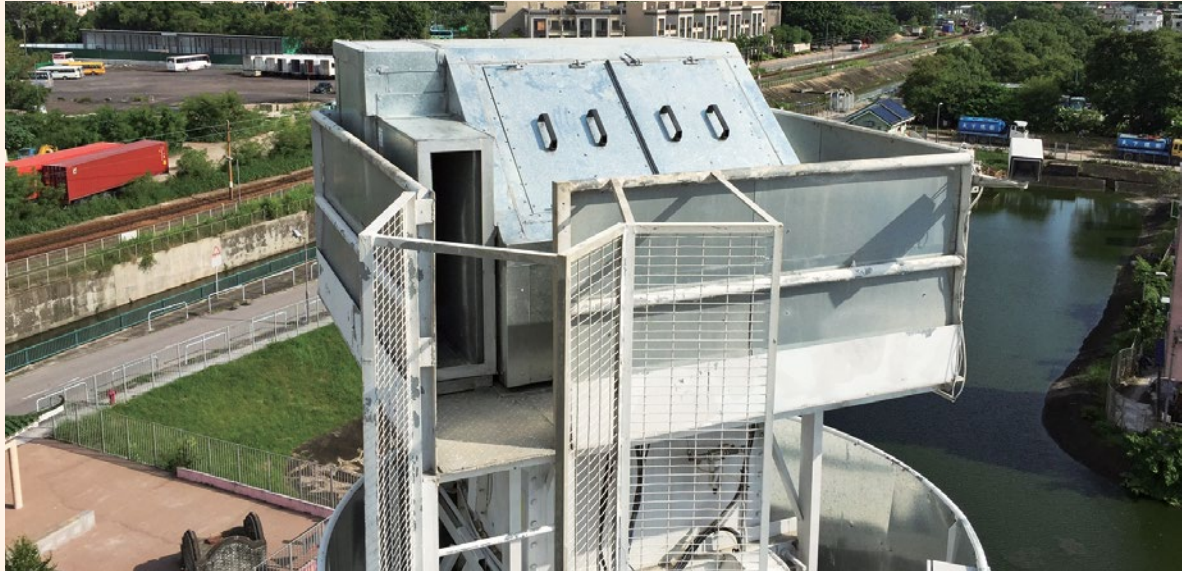
Acoustics enclosure constructed with G.I. high performance sound insulating panels with silencer was installed at the dust collectors reduced the noise transmission to the surrounding area.
