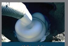
**Light weight**FoamCrete™ is lighter than normal concrete by up to 75%, thus reducing the loading burden and does not impose a lateral load to the
